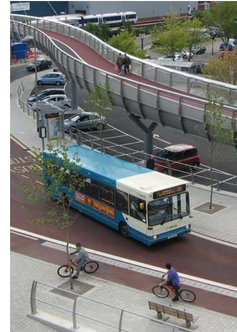
Bourg Walk Bridge
